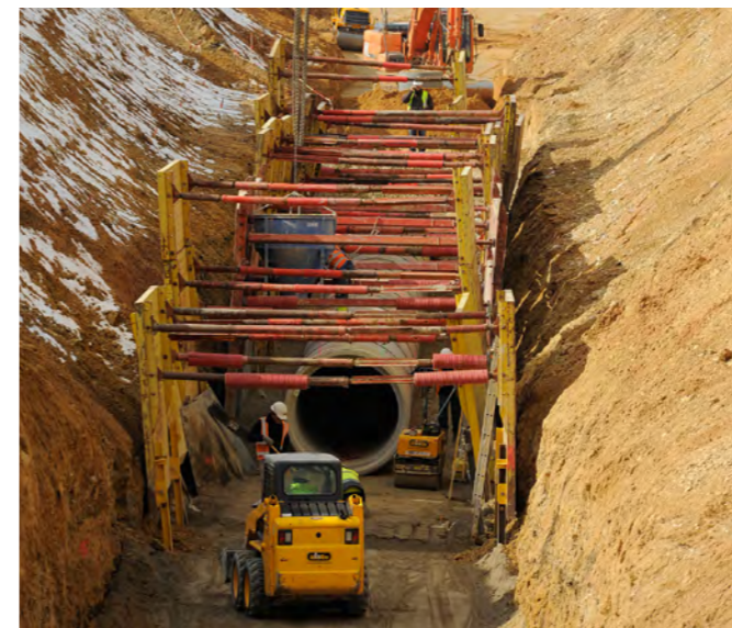
Overflow network-pipes' backfilling
