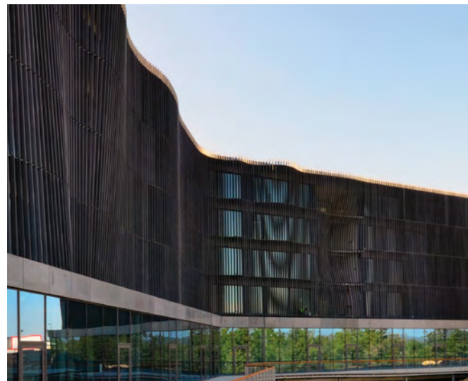
ITER IO Headquarter's building – © ITER IO
