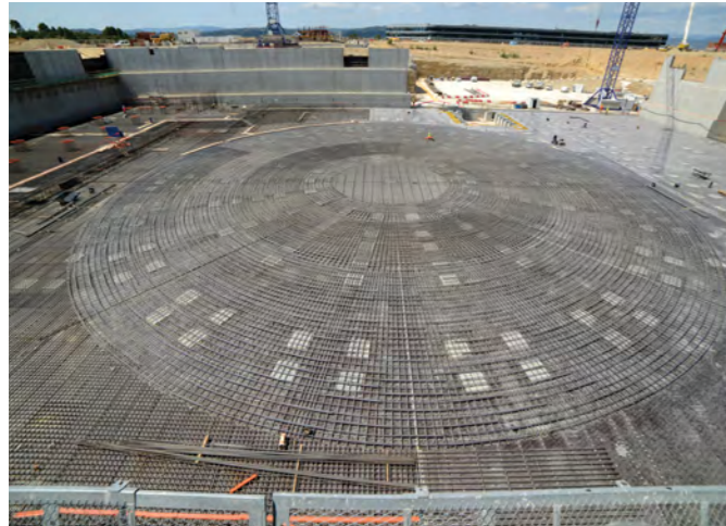
Reinforcement work ongoing (Autumn 2013)
