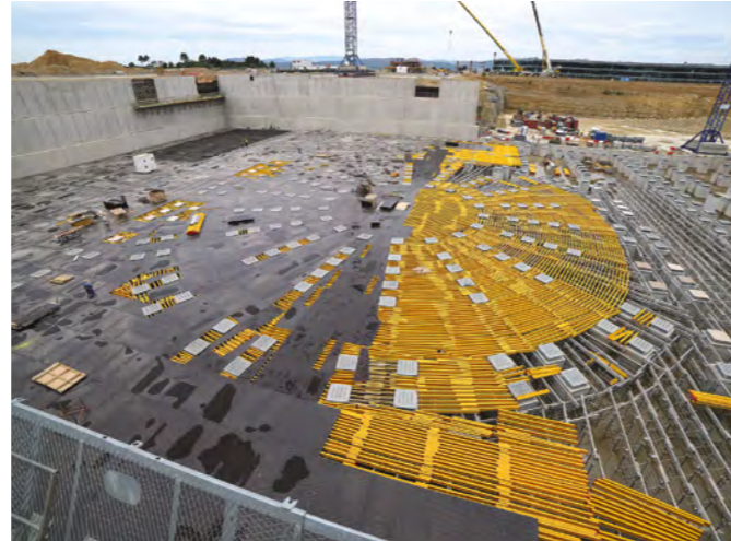
Propping and formwork set up for the upper basemat (Summer 2013)
