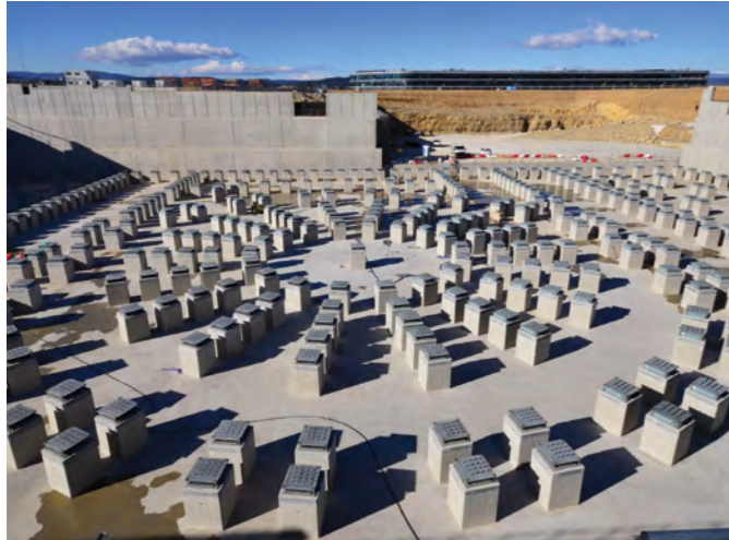
Anti-seismic bearings installed, retaining walls constructed (January 2013)
