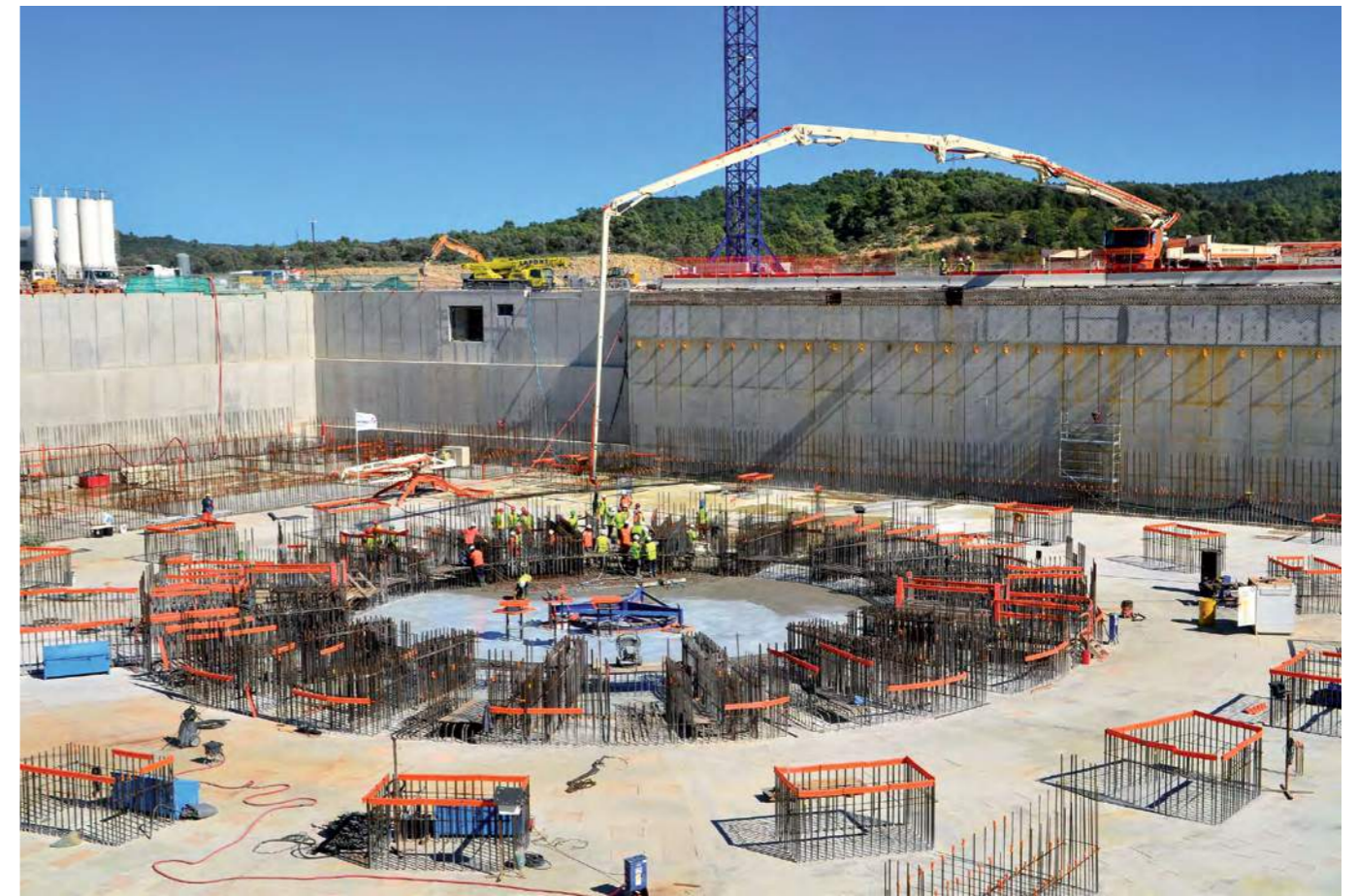
The first floor of the Tokamak complex has been completed
