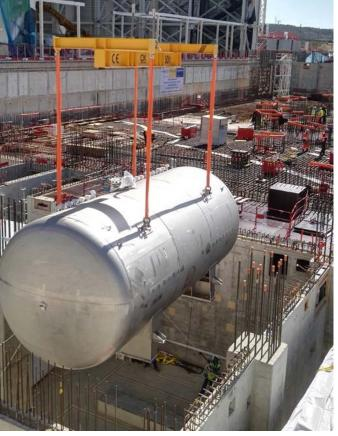
Transferring one of the bigger water detritiation tanks weighing approximately 20 T in ITER's Tritium building
