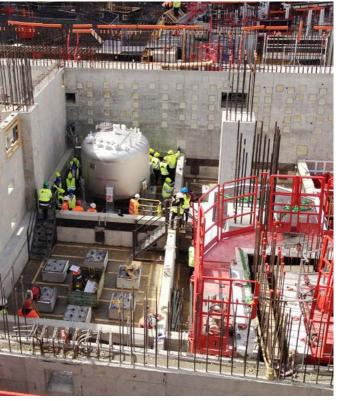
Installing one of the smaller water detritiation tanks in ITER's Tritium building
