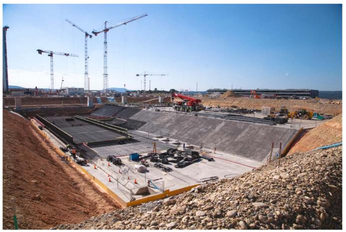
Civil engineering works progressing at the water basin and cooling water stations of the ITER device, November 2016, ITER IO ©
