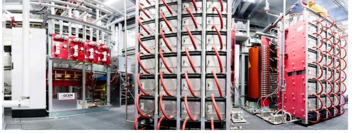
ISEPS of SPIDER equipment fully installed and tested inside the High-Voltage Deck
