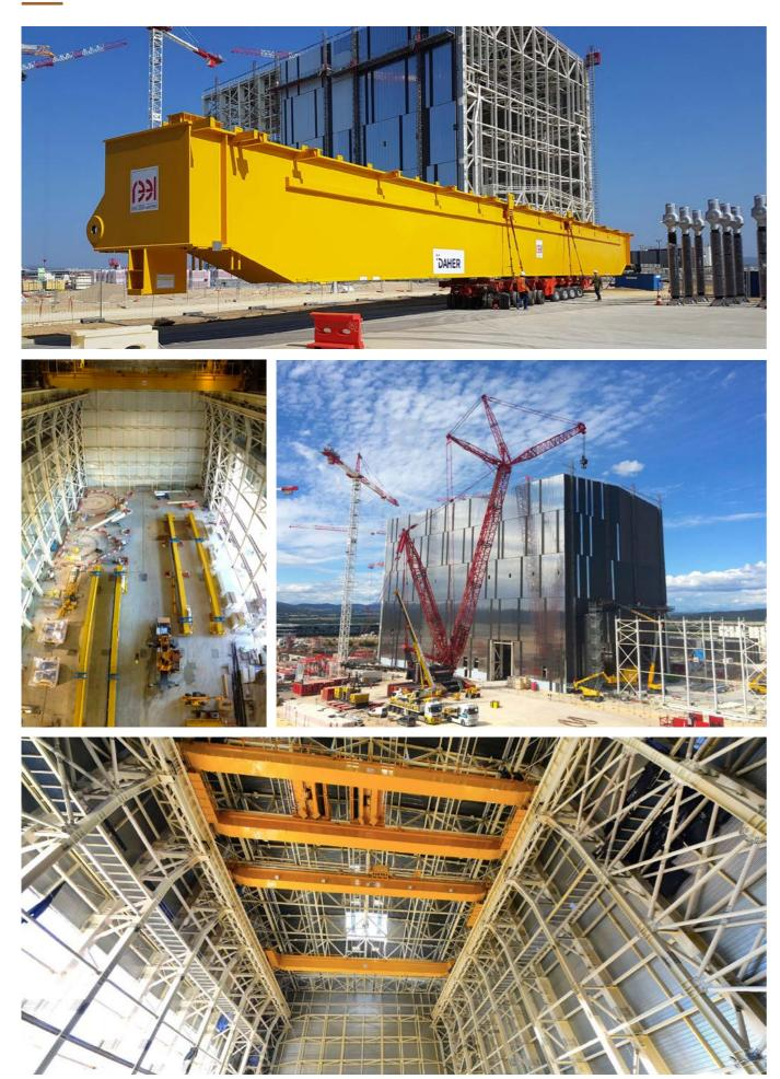
The second girder of the cranes operating in the Assembly Hall has arrived at the ITER site, March 2016 The four girders of the cranes that will lift the bulky ITER components have been installed in the Assembly Hall, July 2016, Cadarache © Engage The impressive monster crawler crane that was used to help with the lifting operation, July 2016, Cadarache The two auxiliary 50 T cranes at the Assembly Hall, November 2016, © Engage
