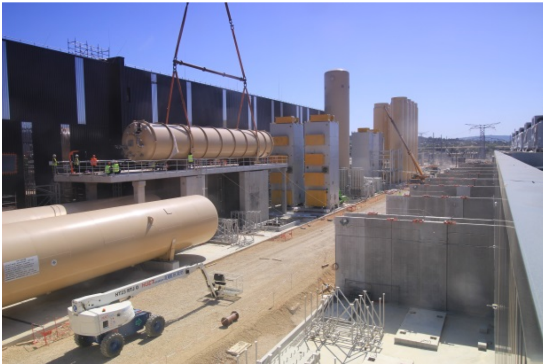
Figure 11: On-site installation of the LN2 Plant and Auxiliary Systems
