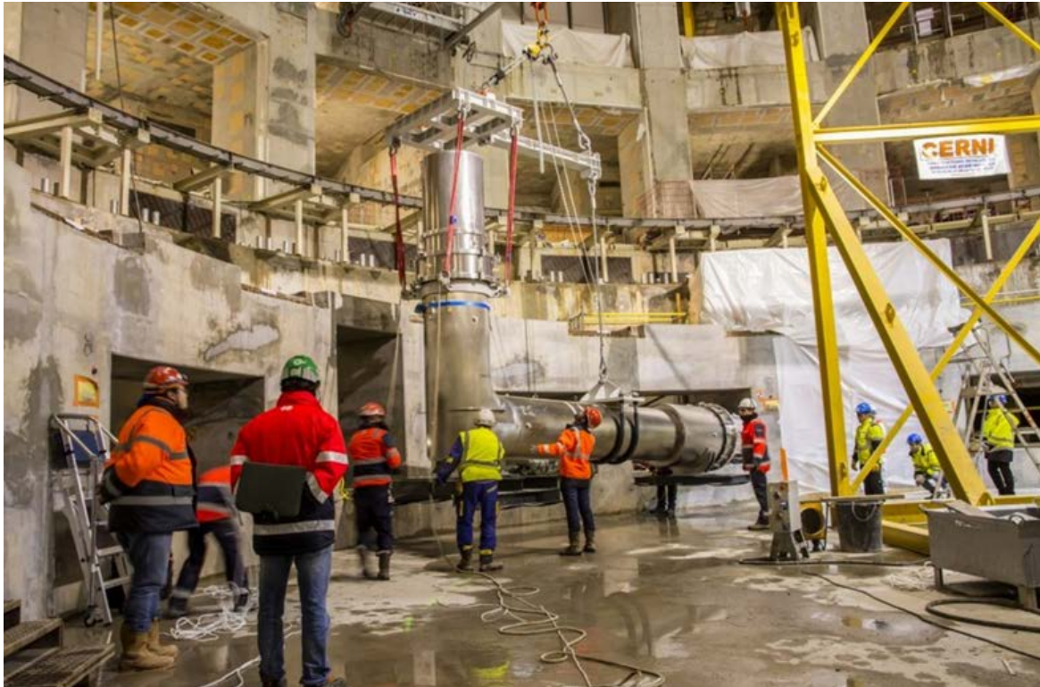
Figure 2: The first machine component, a Poloidal Magnet feeder was introduced in the Tokamak pit (November 2018)
