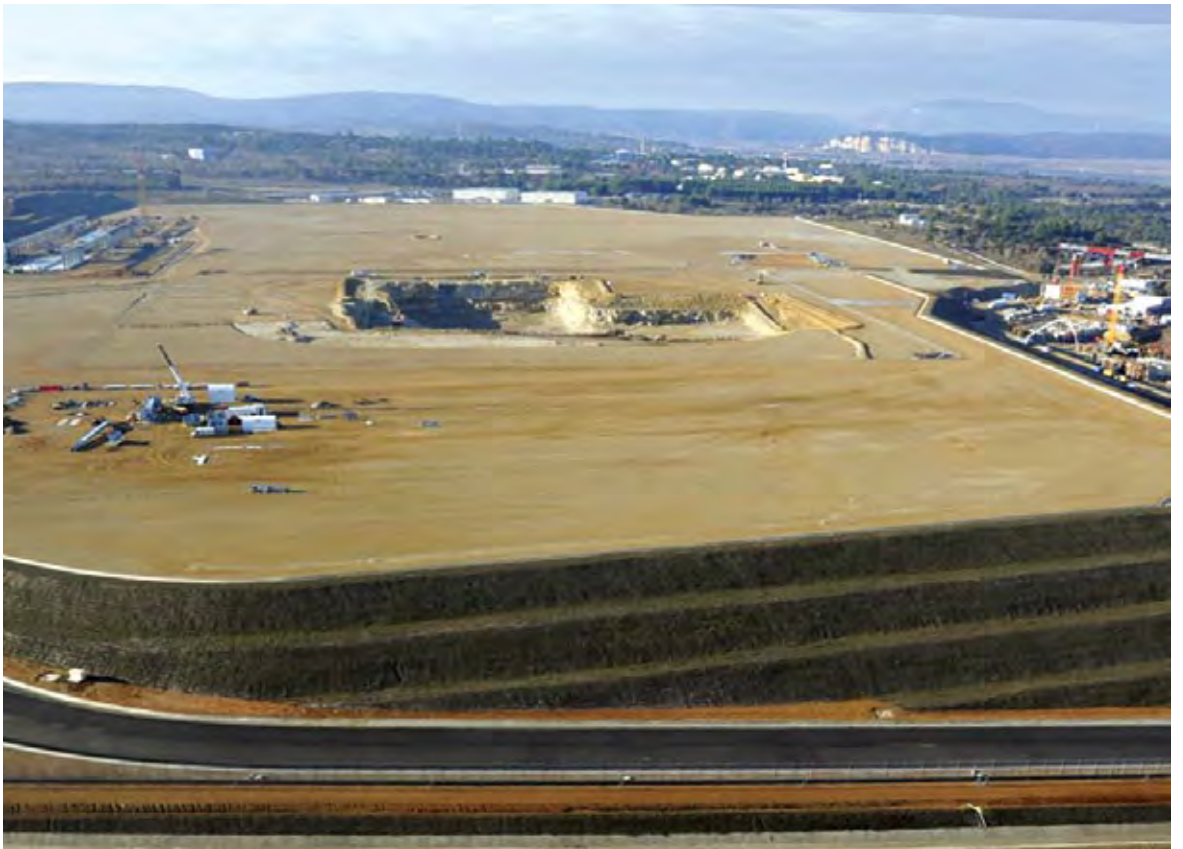
Fig. 22: General view of the ITER Site December 2010 (courtesy of Altivue)
