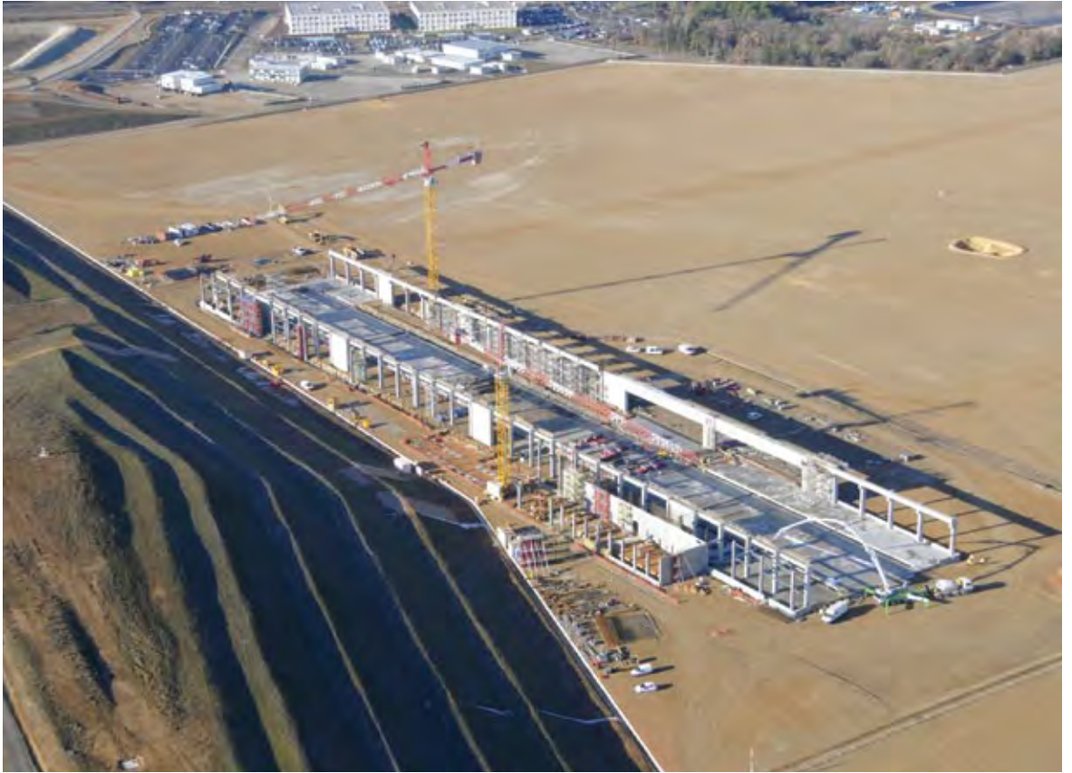
Fig. 21: PF coil building progress December 2010 (courtesy of Altivue)
