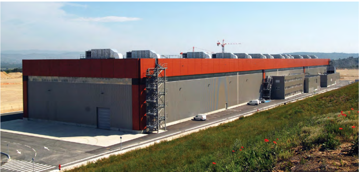
External view of the poloidal field coils building completed, January 2012
