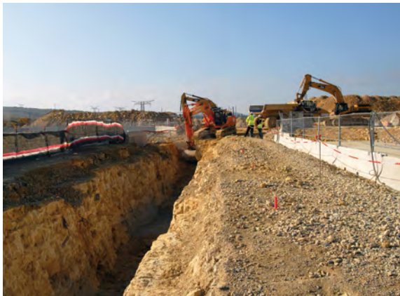
Construction of galleries and tunnels around the tokamak
