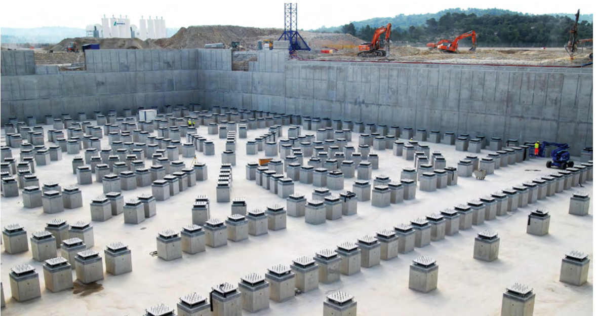
Foundation of the tokamak complex with 493 anti-seismic bearings installed
