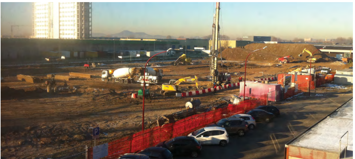
Neutral Beam Test Facility building construction
