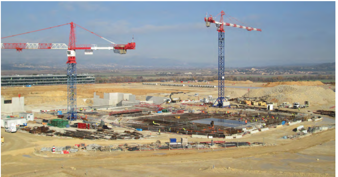
Aerial view of the F4E work site
