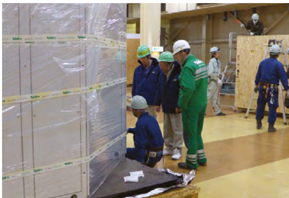
QPC on-site installation activities
