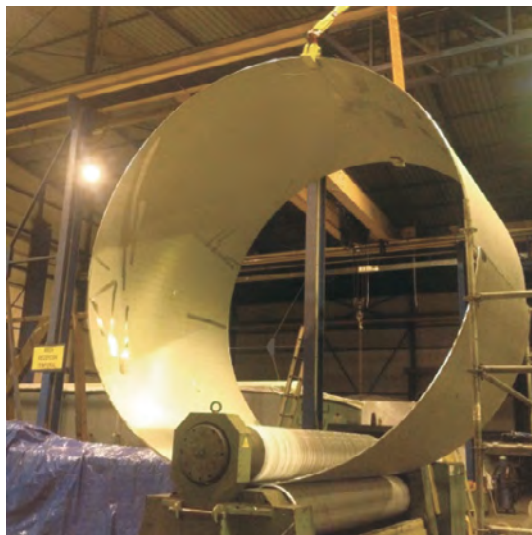
Cold forming of 100 m³ tank shell sector.
