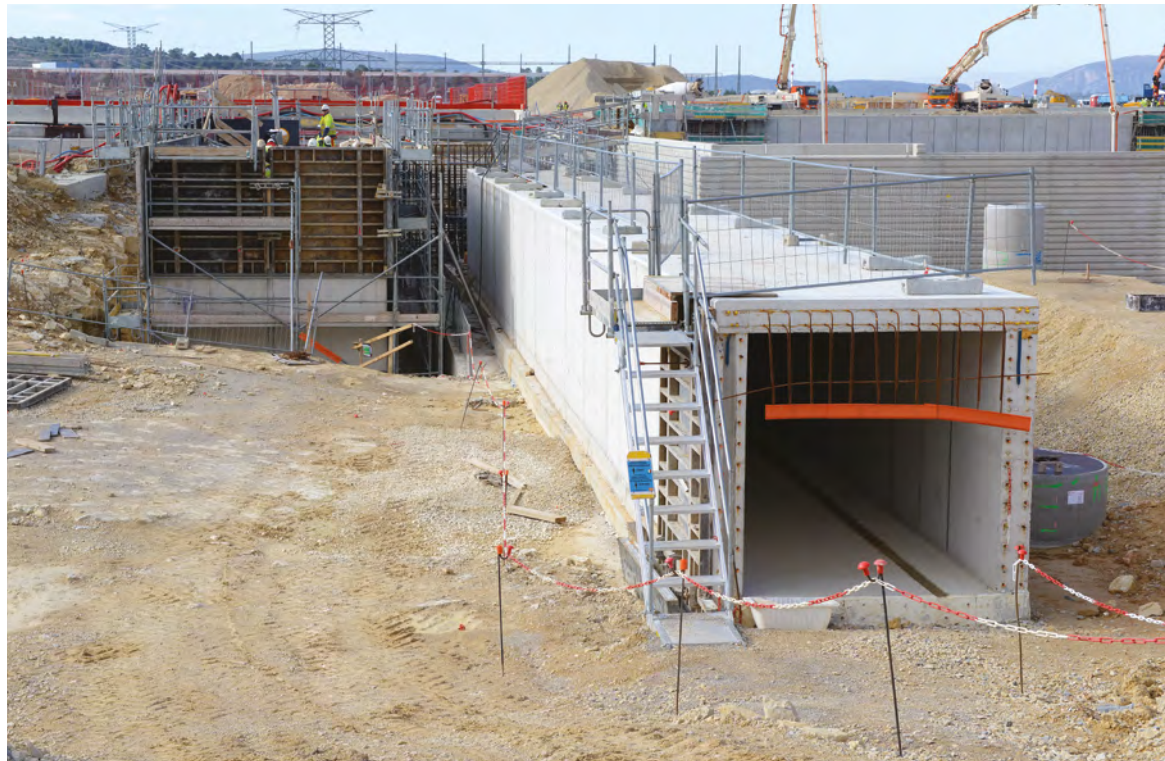
Galleries in the vicinity of the Tokamak Complex
