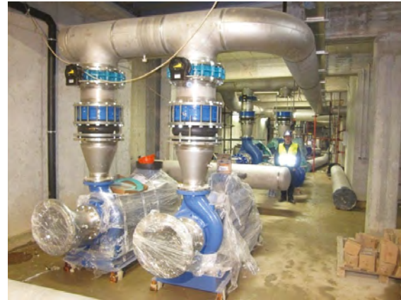
NBTF cooling plant on-site installation
