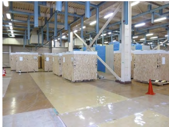
QPC components stored in the rectifier building
