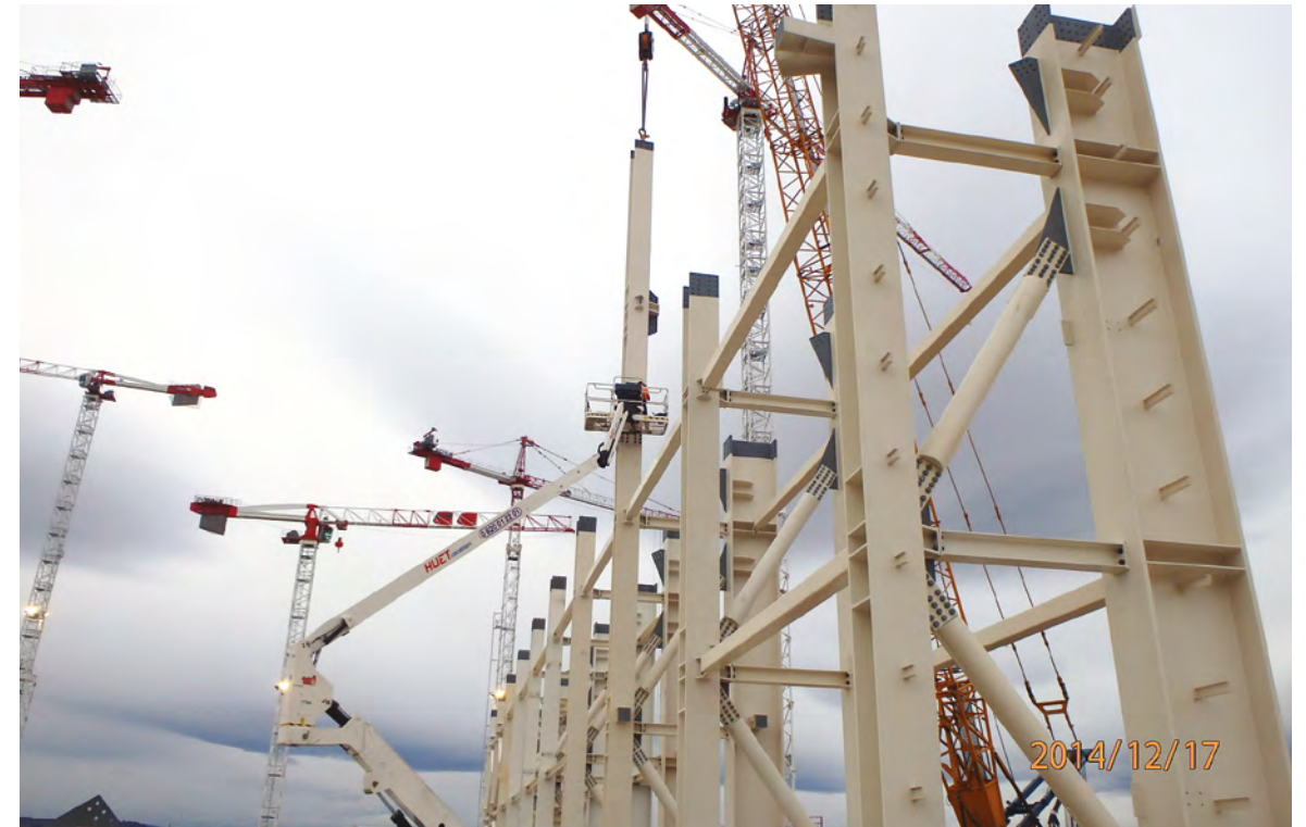
Start of steel works at the Assembly Hall building
