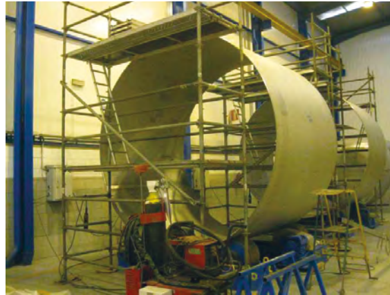
Welding of shells of 20 m³ tank.
