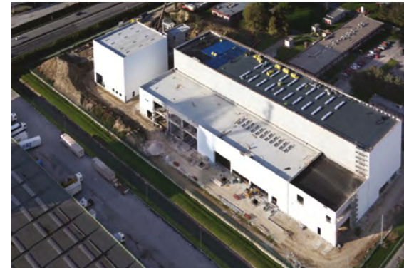
NBTF building under construction at the Padua site (Consorzio RFX premises)
