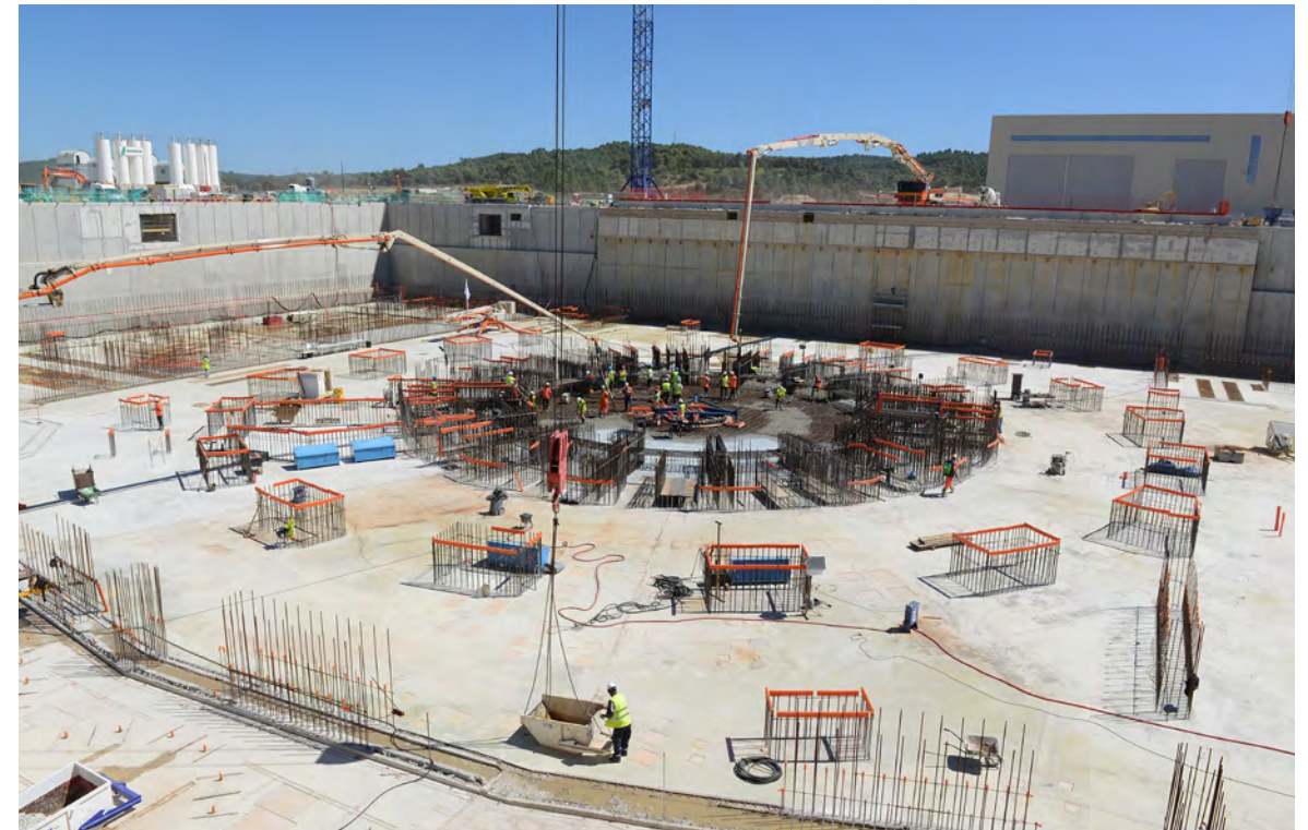
Completion of the first floor slab of the Tokamak Complex
