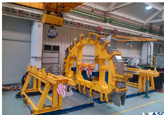
Coil 1 – welding of casing after coil insertion (September 2015) (Courtesy ASG/ENEA).
