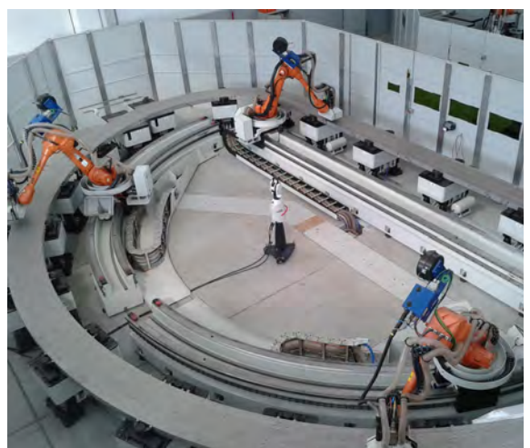
The laser welding machine in operation during welding of cover plates on a regular DP in ASG, La Spezia
