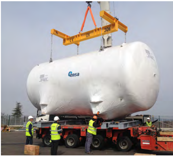
Delivery at ITER site of a 100 m 3 tank
