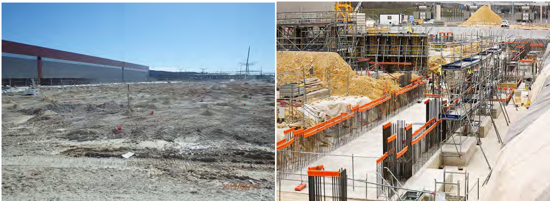
The Cryoplant buildings in March 2015 and in December 2015
