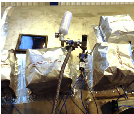
Helium leak test of 100 m 3 tank
