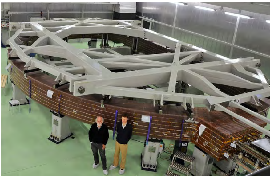
Series DPs, stacked together to form the first ITER TF coil Winding Pack in ASG, La Spezia (Courtesy of ASG)
