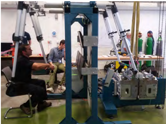
RH cutting/welding tests in the full-scale mock-up for NB pipelines and bellows
