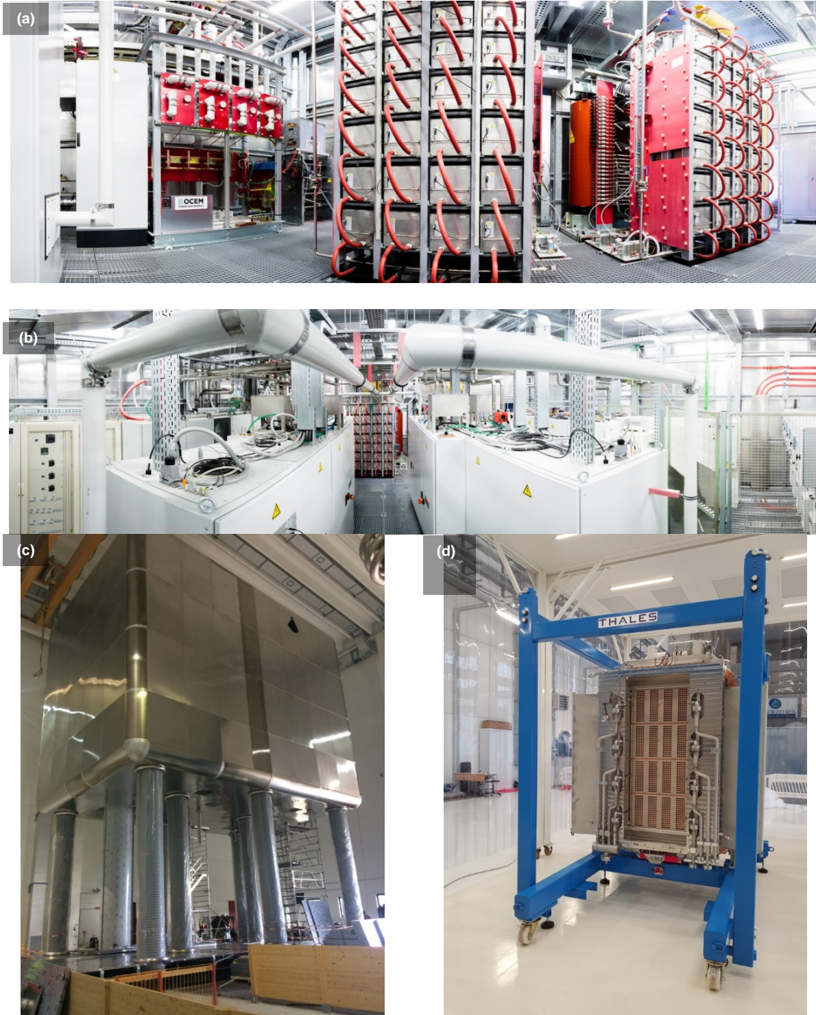
Figure 13: Progress at the Neutral Beam Test Facility in Padua, Italy including (a-b) the SPIDER Ion Source and Extraction Power Supplies installed inside the High Voltage Deck, (c) the outside of the High Voltage Deck and Bushing and (d) the SPIDER Beam Source
