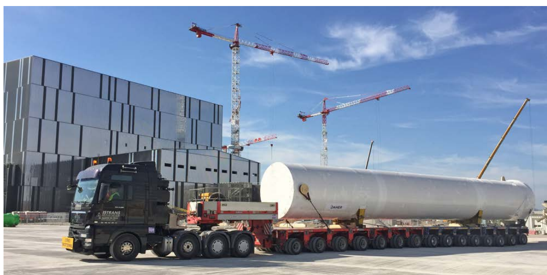
Figure 12: The gaseous liquid nitrogen tank, part of ITER’s cryogenic system, being delivered to ITER
