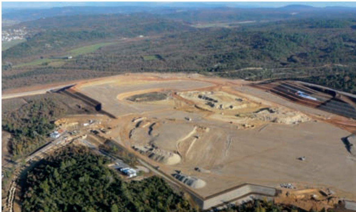
ITER construction site: site levelling completed. (AIF©)
