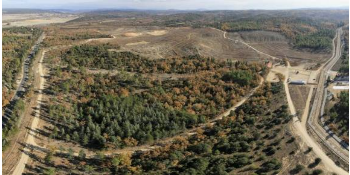
Figure 9 – ITER Platform beginning 2008
