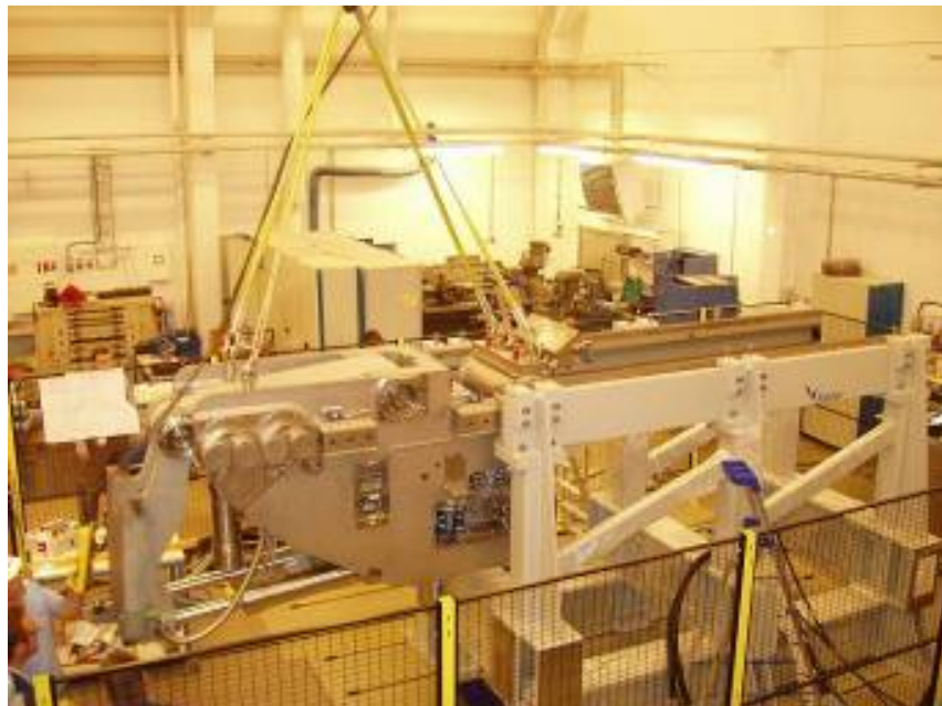
Figure 26 - Installation of the Cassette Multifunctional Mover prototype in the test stand in DTP2 - Finland
