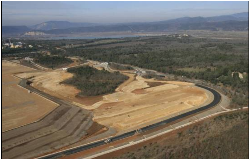
Figure 12 - Earthworks for Annex Buildings
