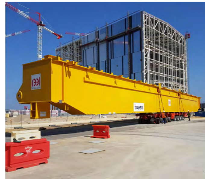
The second girder of the cranes operating in the Assembly Hall has arrived at the ITER site (left) and in the Marseille industrial harbour of Fos-sur-Mer, March 2016.
