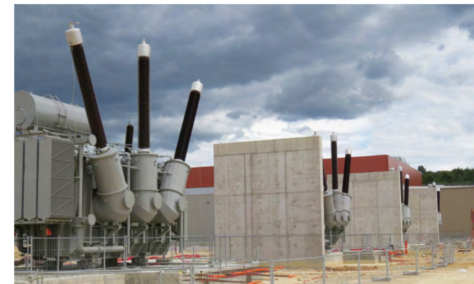
Work progressing at the Transformers area, ITER construction site, June 2016 © F4E
