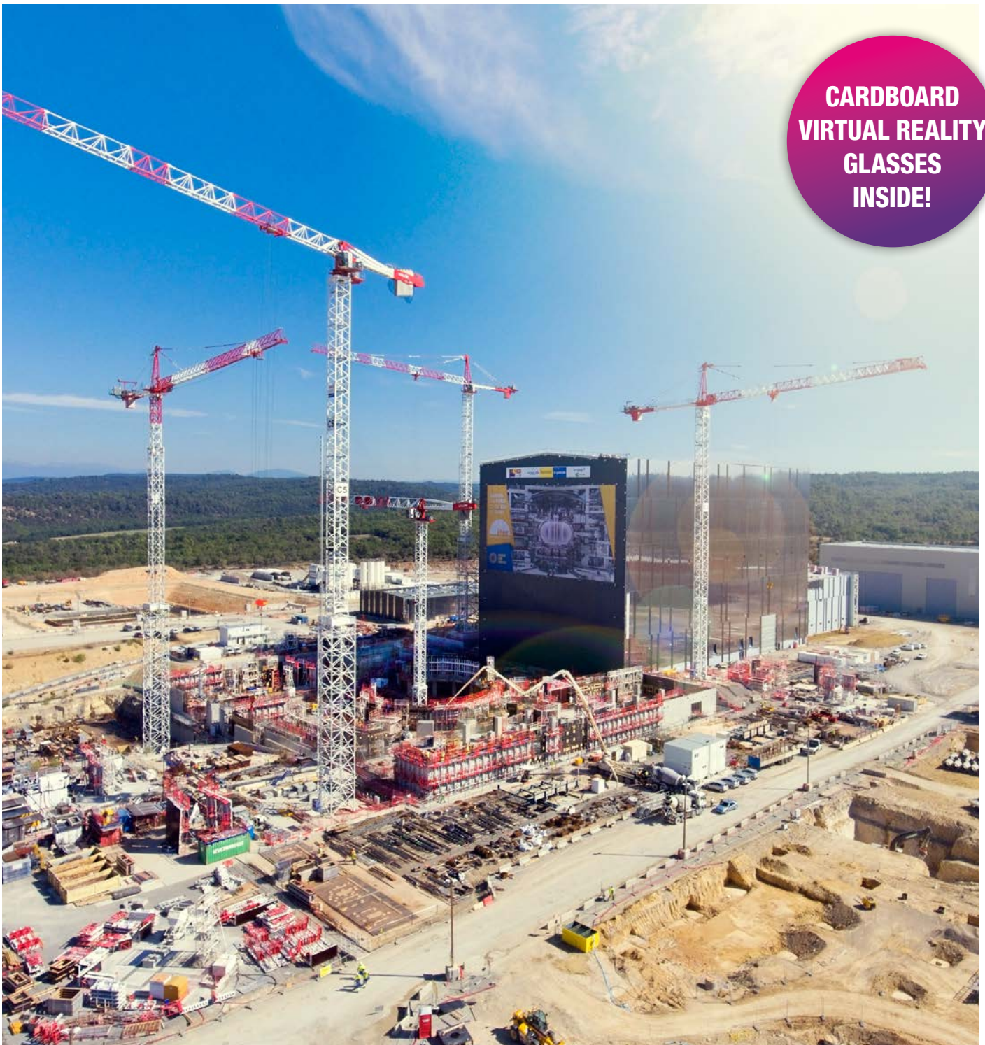
ITER construction site - October 2016
