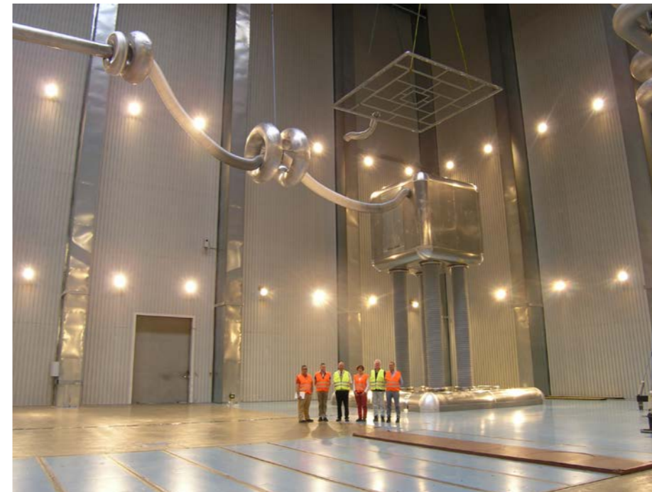
The testing team at the High Voltage Laboratory at HSP GmbH © Siemens AG, 2016. All rights reserved.
