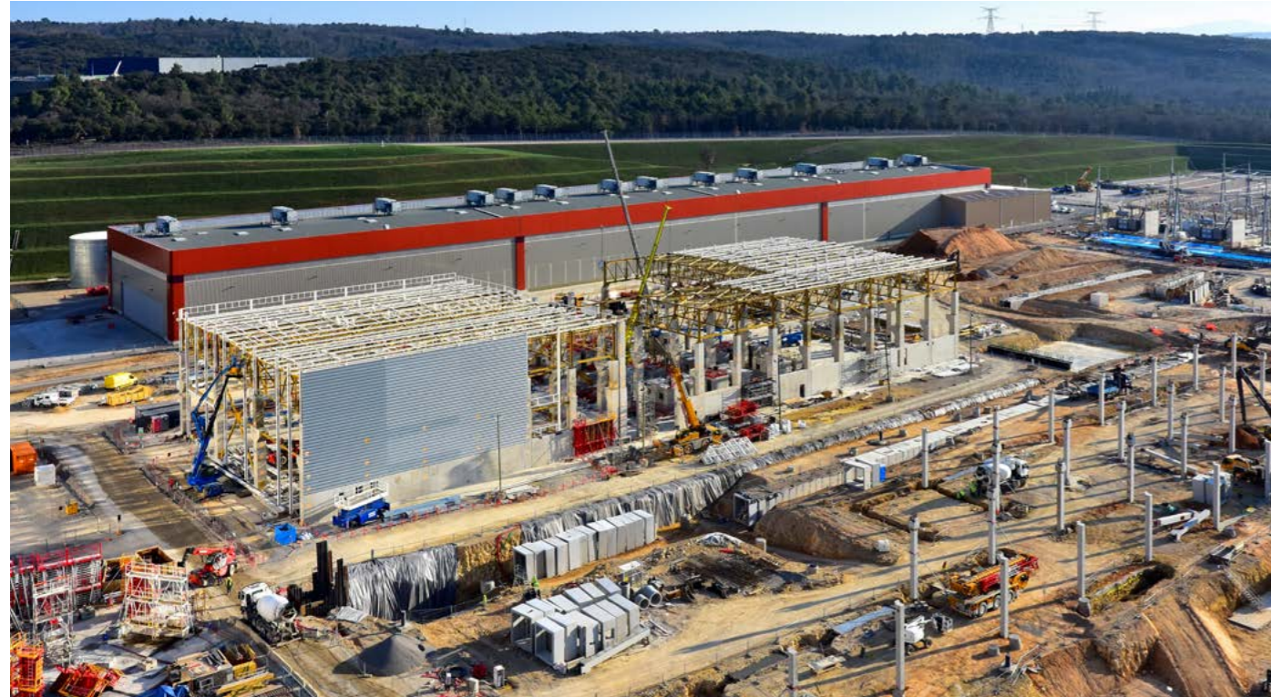
Construction in progress at the Cryoplat facility, April 2017, © E. Riche/ITER Organization
