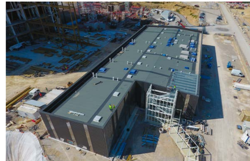
Aerial view of the Site Services building, September 2016, © LNM
