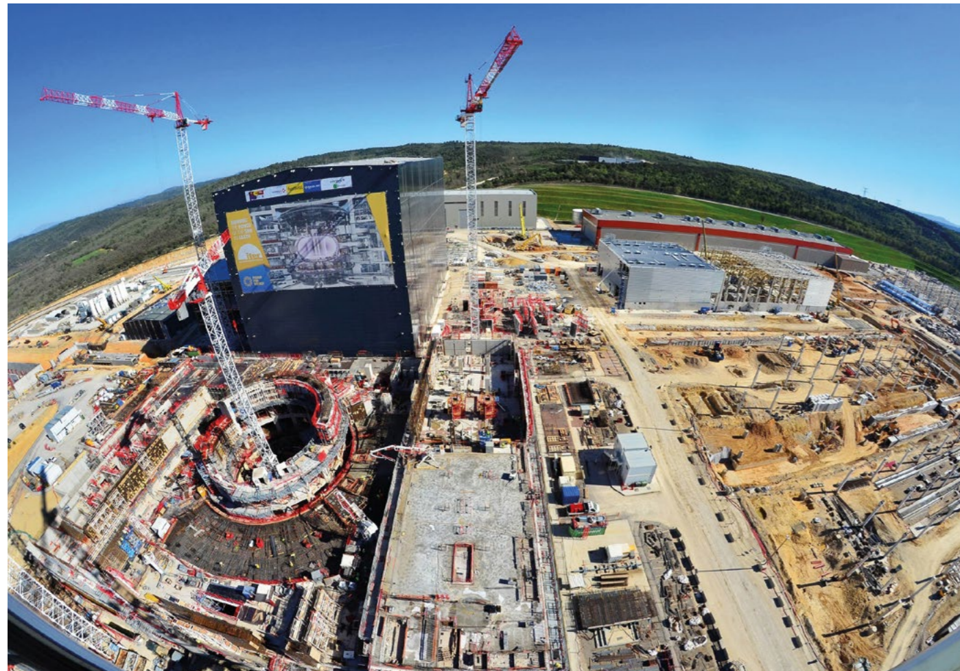
ITER construction site, April 2017, © ITER IO
