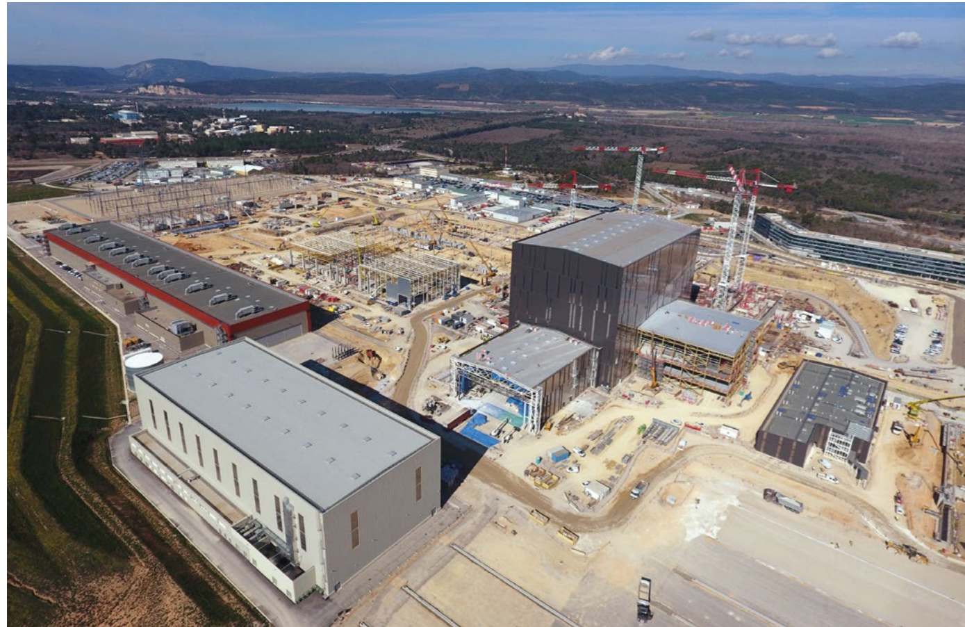
The impressive ITER Assembly Hall (dark metallic structure) and Site Services buildings (adjacent to the right), April 2017 © Engage
