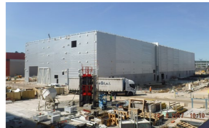
The Cryoplant facility under construction, ITER construction site, Cadarache, June 2017 © Engage
