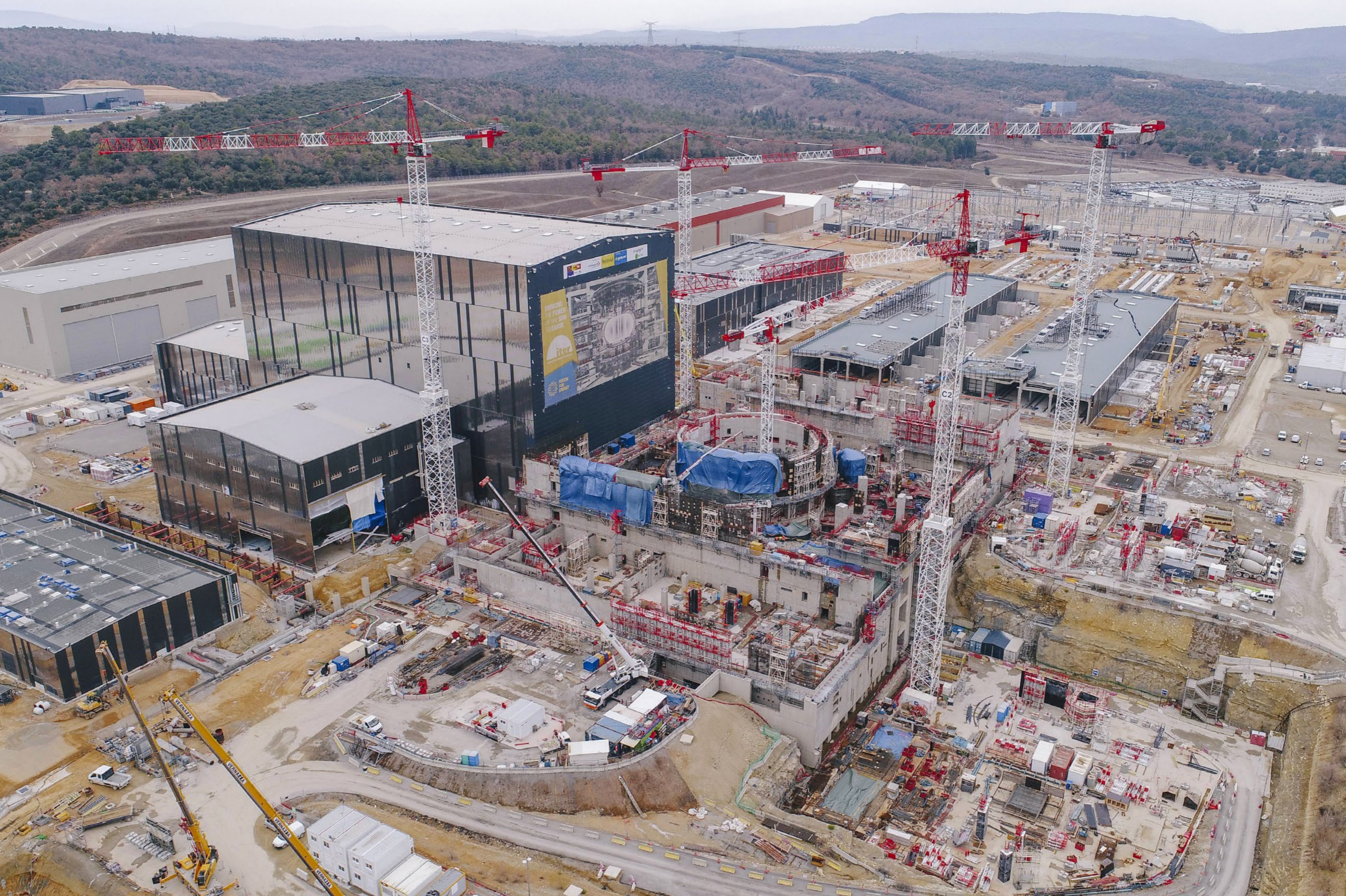
Aerial view of the ITER worksite December 2017 © SNC Engage
