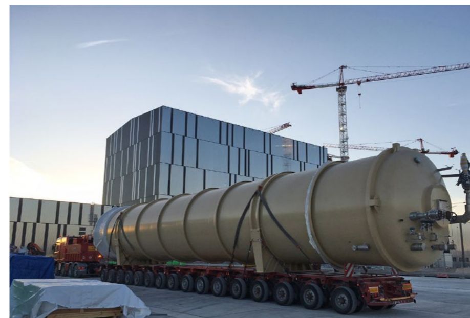
The LHe tank, widely considered as the "jewel" of the ITER Cryoplant, has finally reached the construction site, Cadarache, October 2017 © DAHER
