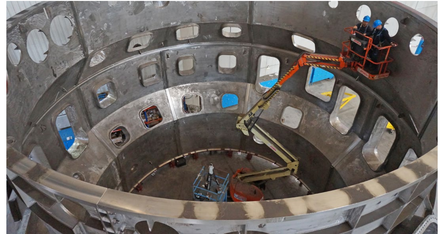
The cryostat vessel body seen from above.
