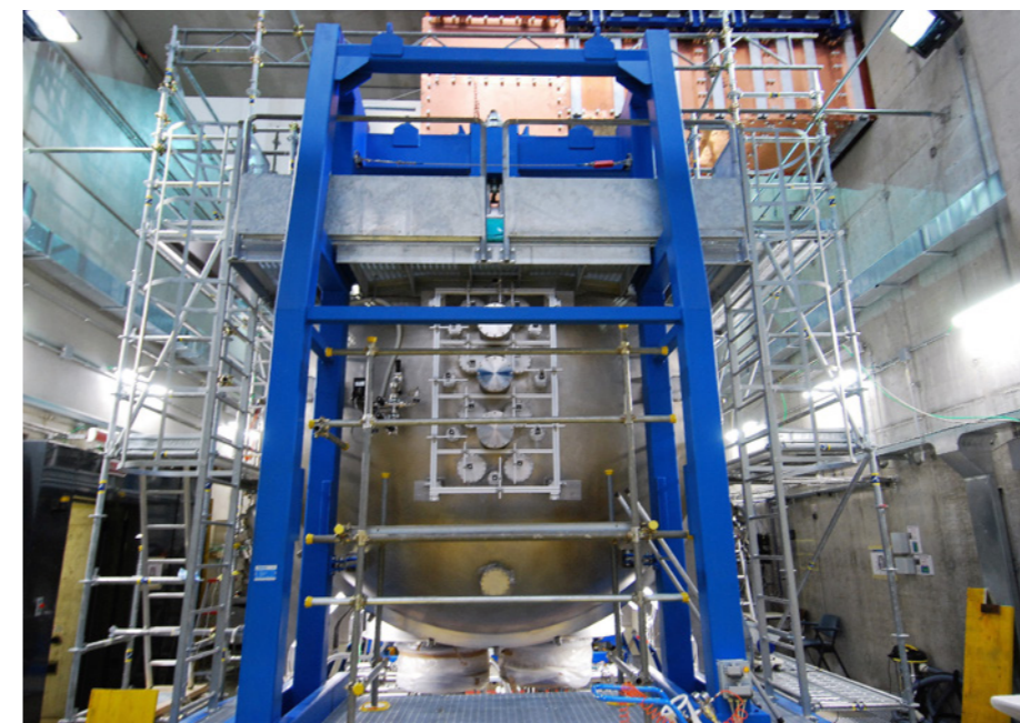
Getting ready to lock the SPIDER beam source in its vessel, ITER Neutral Beam Test Facility, Consorzio RFX, Padua, Italy
