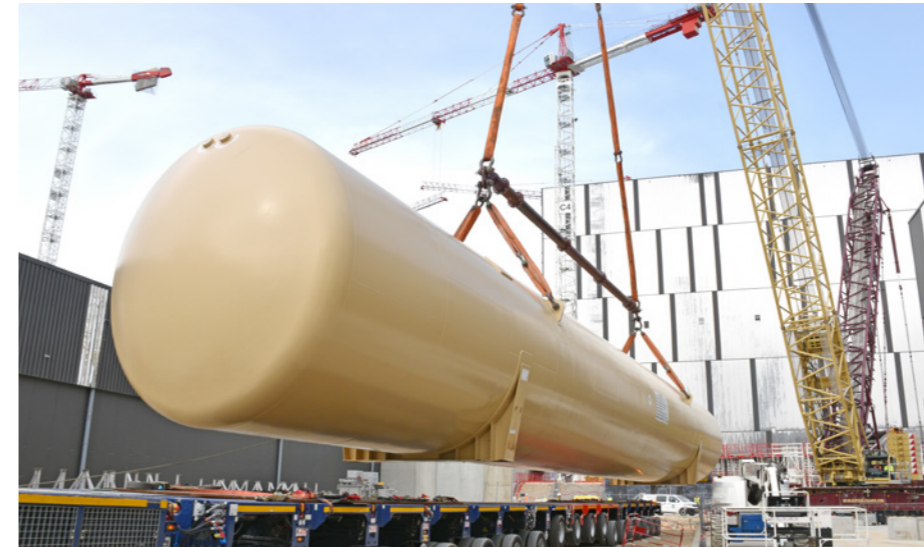
Lifting one of the two quench tanks financed by F4E and produced by Chart Ferro. ITER Cryoplat, April 2018.
