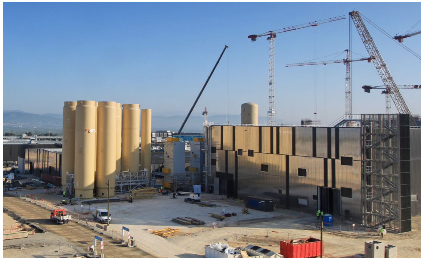
Finalising the installation of Europe's cryogenic tanks on-site, ITER Cryoplat, April 2018.
