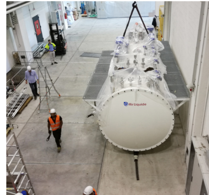
Unpacking the auxiliary cold box at the ITER Neutral Beam Test Facility, MITICA, Padua, Italy
