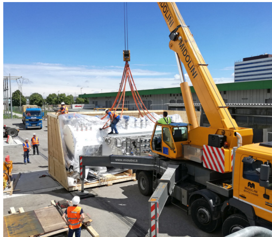
Unpacking the auxiliary cold box at the ITER Neutral Beam Test Facility, MITICA, Padua, Italy
