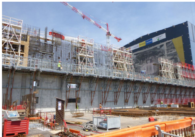
Tokamak Building Level 5 construction on-going, ITER construction site, Cadarache, June 2018
