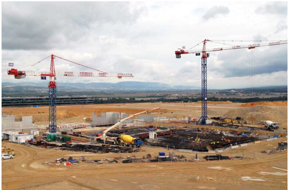
Works in progress at the ITER Tokamak Assembly Hall, October 2012
