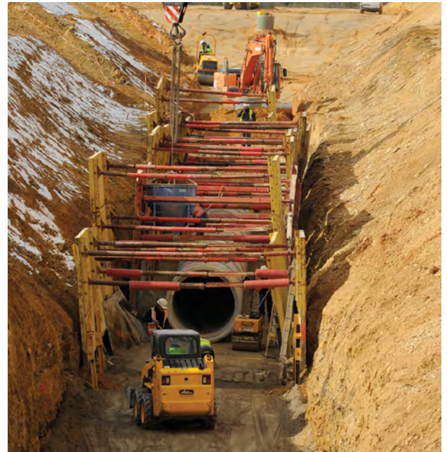
Overflow network - pipes' backfilling
