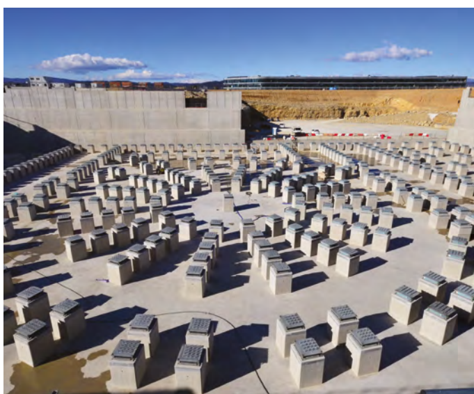
From plinths to full basemat: four key stages of the ITER Tokamak basemat
