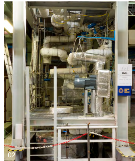
02 ITER Test Blanket Modules - ENEA, Brasimone, Italy - IELLLO, one of the biggest forced circulation Lead Lithium Loops in Europe
