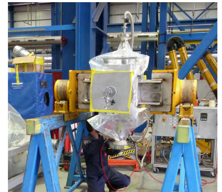
Heatric technical staff carrying out the helium leak test.
