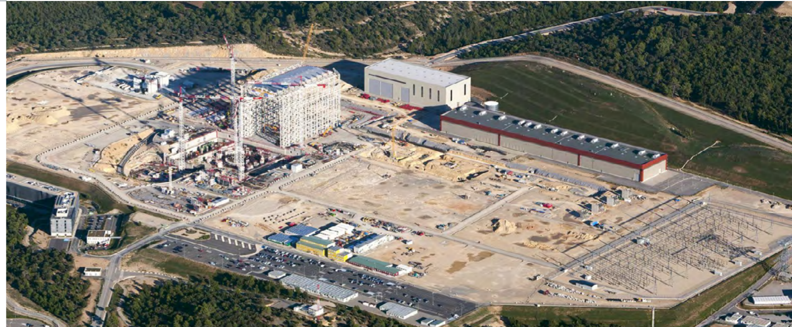
Aerial view of the ITER construction site, October 2015 © Matthieu Colin.com
