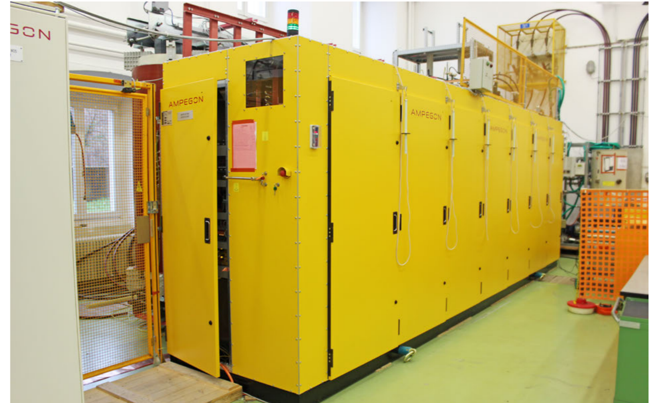
High Voltage Power supply unit procured by F4E and manufactured by Ampegon © Fusion for Energy
