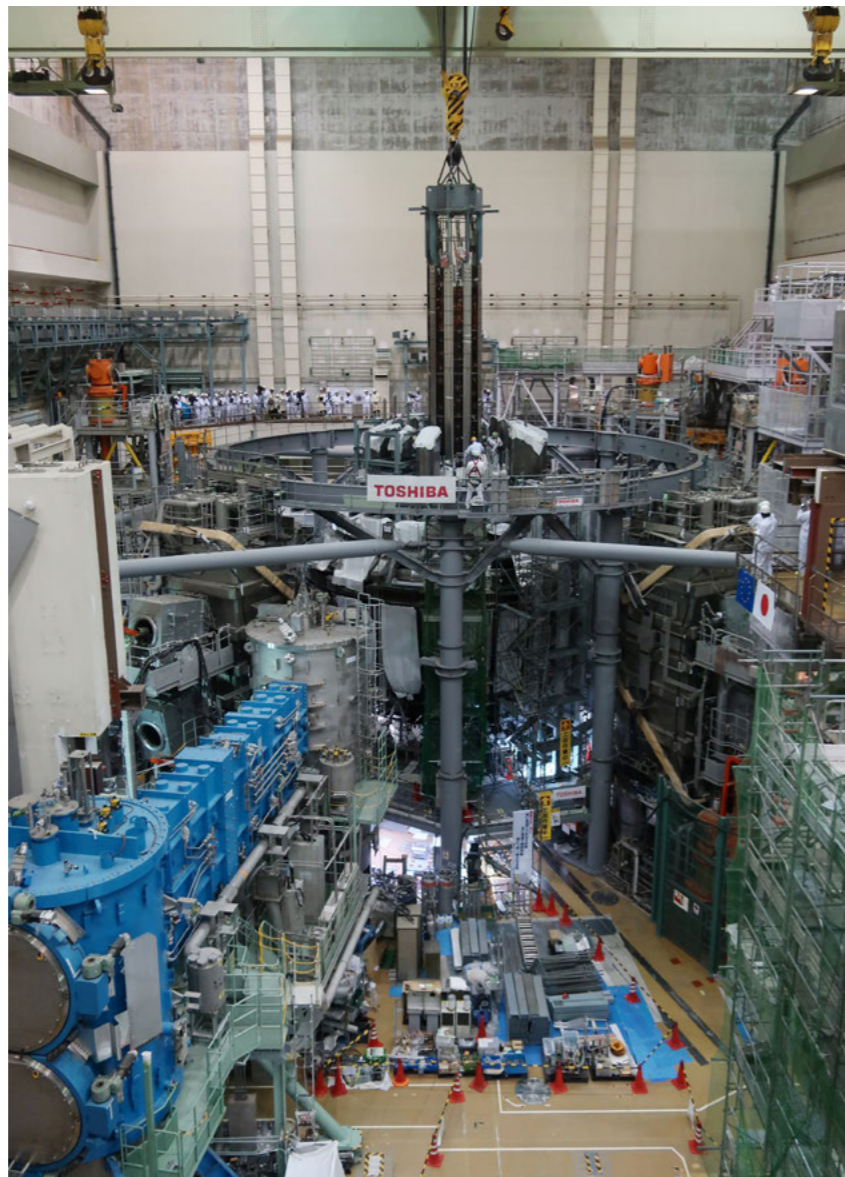
View of the JT60-SA as operation insertion of the central solenoid advances, Naka, Japan, May 2019
