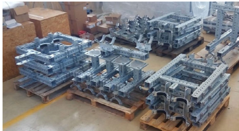
Delivery of the supports of the warm regeneration lines
