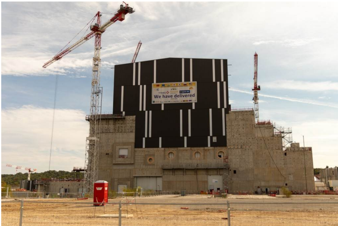
Figure 1: The ITER construction site showing the Tokamak Complex.
