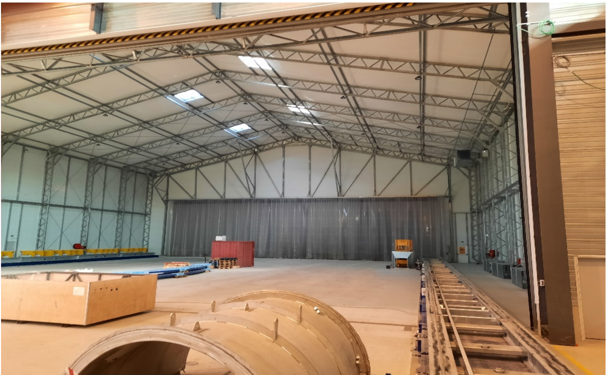
Figure 12: Poloidal Field Coil Workshop extension completion in Cadarache.
