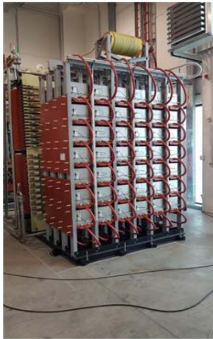
Figure 33: MITICA Acceleration Grids PS Conversion system (AGPS-CS)
