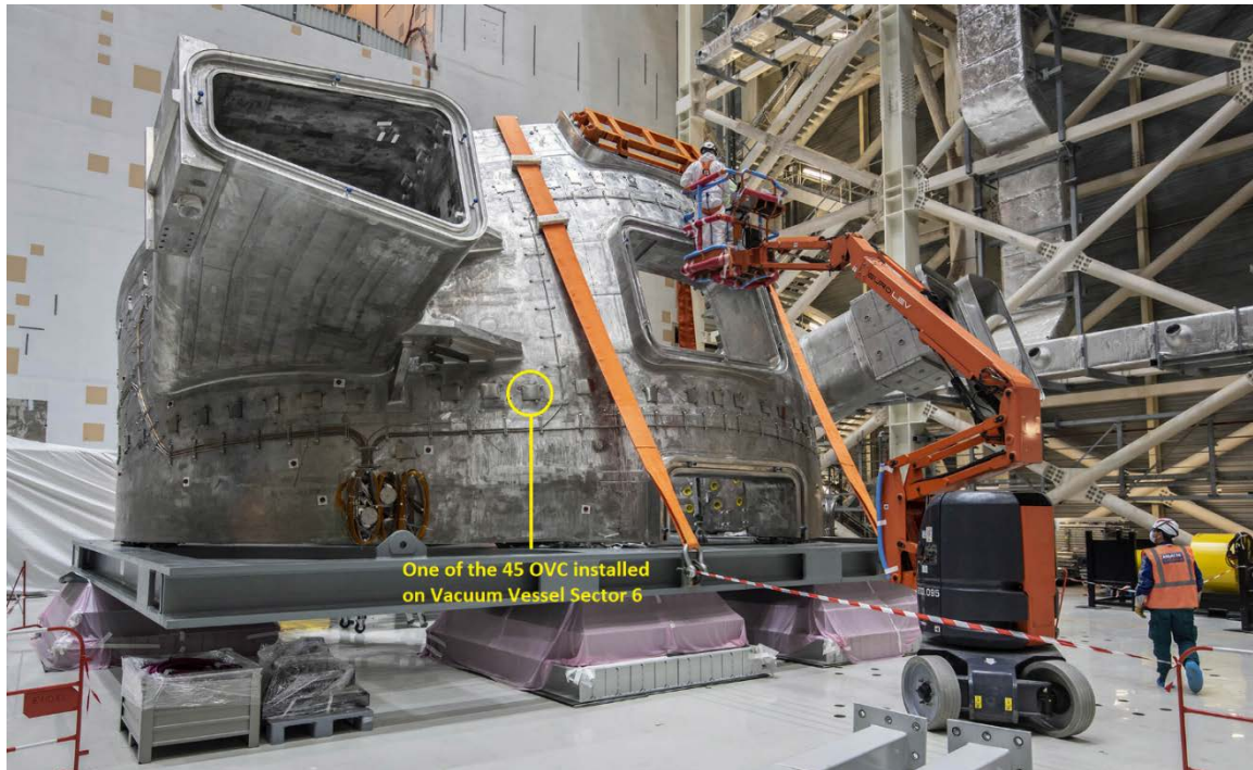
Figure 24: One of the 45 OVC installed on Vacuum Vessel Sector 6
