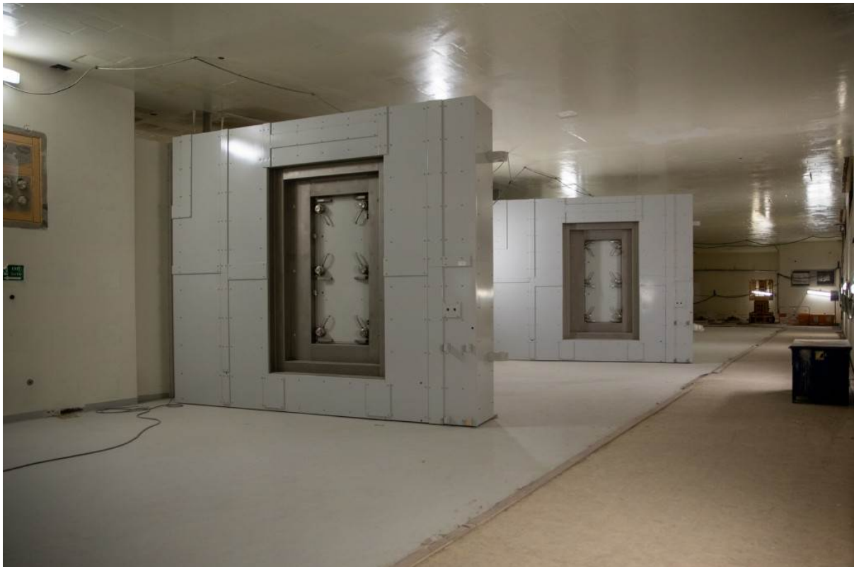
Figure 3: Tokamak Building (B11) All port Cell Doors Installed
