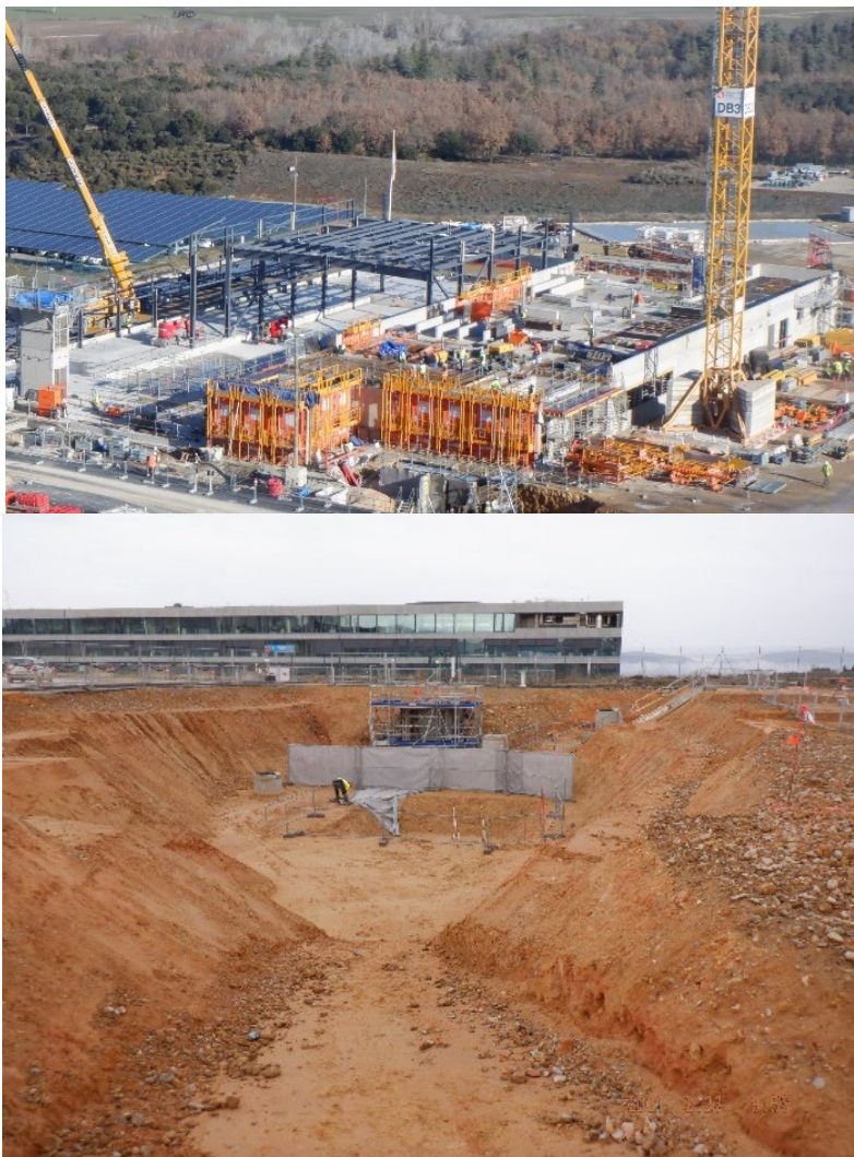
Figure 4: TB12 (Demathieu Bard) B71 North work status in Early 2021 versus December 2021
