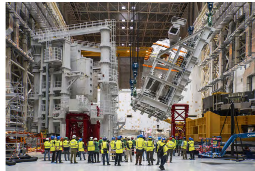
A 90° tilt in mid-air for the first vacuum vessel sector upended, March 2021 © ITER Organization
