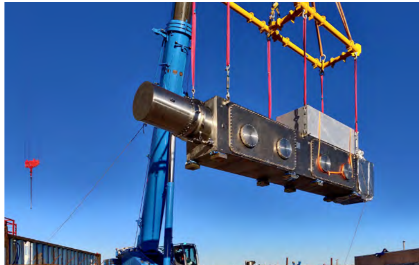
Magnet terminal box, procured by China and manufactured at the Institute of Plasma Physics, Chinese Academy of Sciences (ASIPP), lifted and moved inside the basement of the Tokamak Building. January 2021 © ITER Organization
