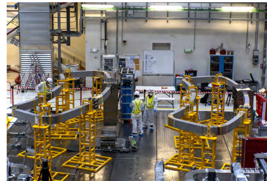
Acceptance tests of correction coils, procured by China, completed successfully. October 2021 © ITER Organization
