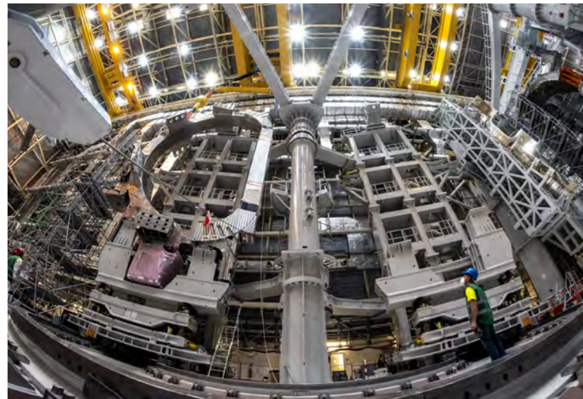
First Toroidal Field coil positioned on tool, June 2021 © ITER Organization
