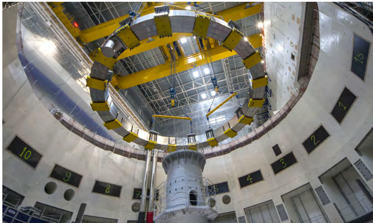
Europe's fifth Poloidal Field coil successfully descends in the Tokamak pit. Cadarache, France, September 2021. © ITER Organization
