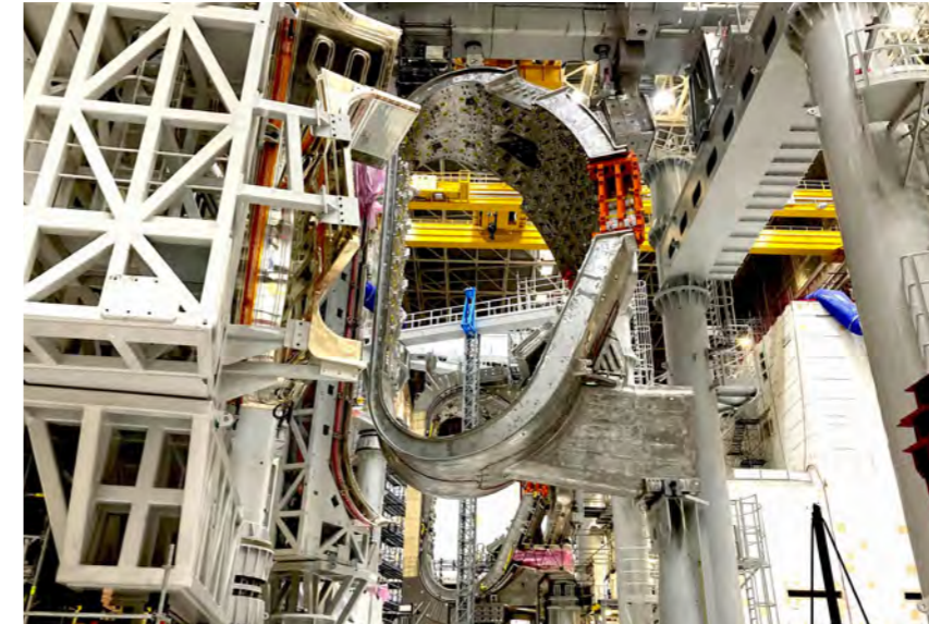
Second vacuum vessel sector positioned on assembly tool, December 2021 © ITER Organization
