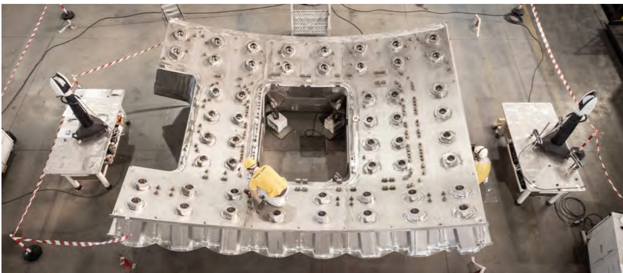
Technicians performing dimensional checks on Europe's vacuum vessel sector 4, poloidal segment 3, Walter Tosto, Italy, December 2021. © Walter Tosto
