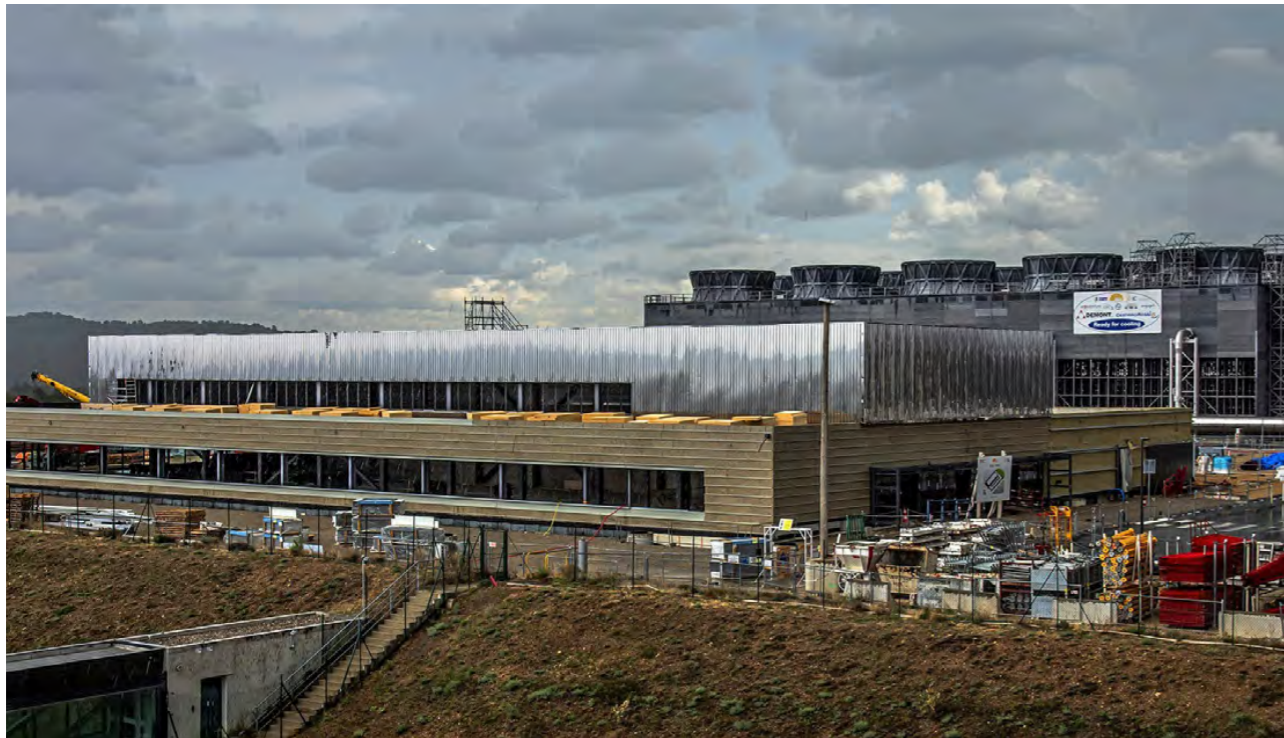
View of the ITER Control Building, connected under the ground with ITER Organization Headquarters, ITER Construction site, Cadarache, France, September 2022 © ITER Organization
