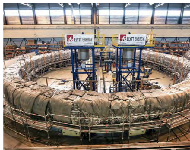
In July, contractors to the European Domestic Agency carry out the vacuum pressure impregnation (VPI) of poloidal field coil #4. July 2022. ©ITER Organization
