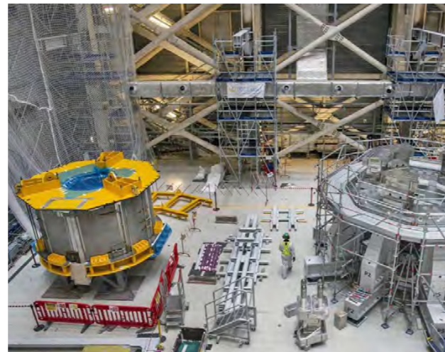
First ITER central solenoid module to enter assembly process. February 2022. ©ITER Organization
