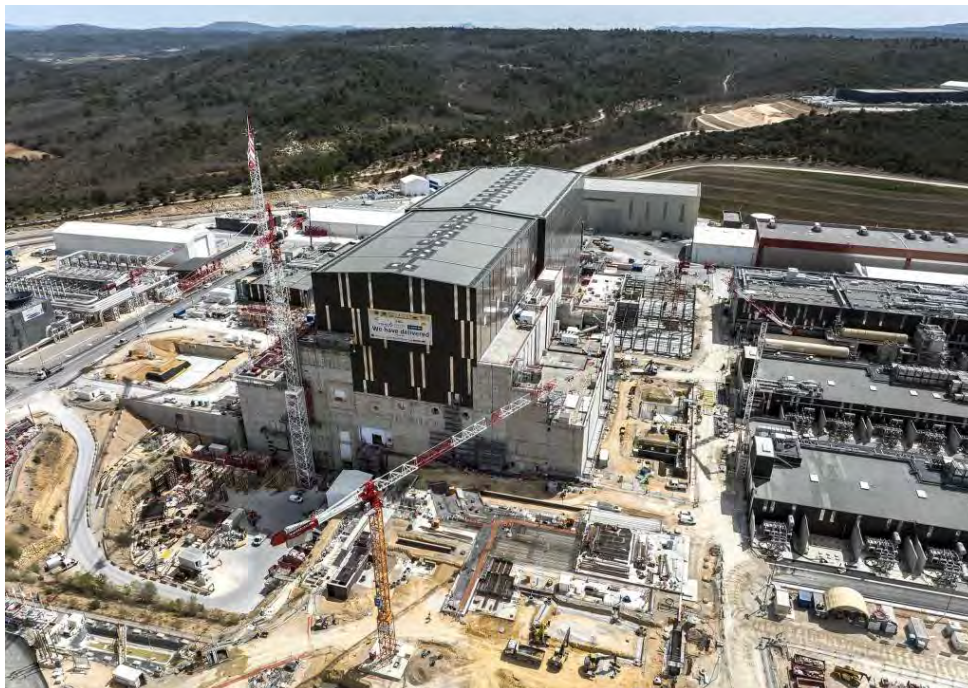
Figure 1: Aerial view of the ITER construction site. Photo: ITER Organization (April 2022)
