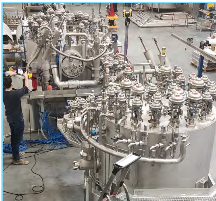
Figure 21: 2 of the 4 cold valve boxes ready to be delivered
