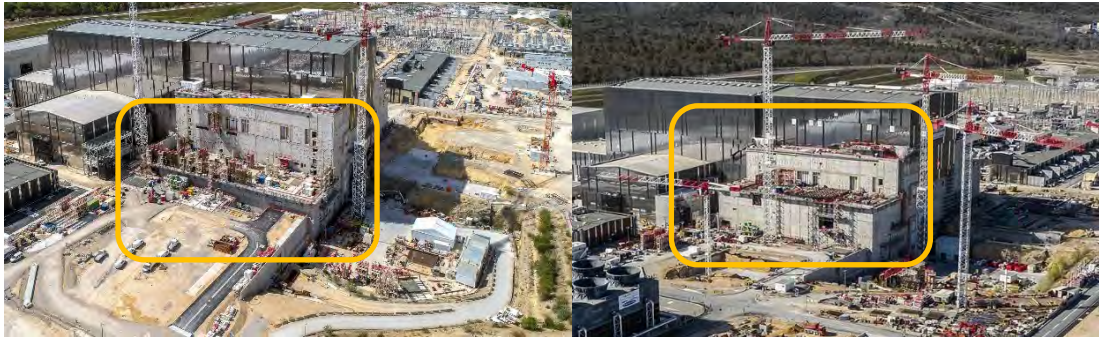
Figure 2: TB18 (Vinci-Ferrovial-Razel, VFR) B14 Tritium Building work status in May 2021 (left) versus April 2022 (right) Photos: © ITER Organization
